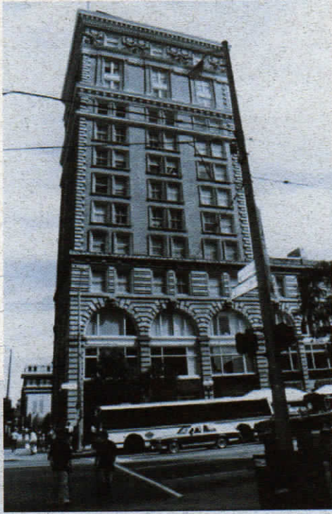
The American Building will serve as the RTA's downtown transit hub, administrative offices, customer waiting facility and as a transit-compatible link to the RTA Center located in the downtown Marketplace Transit Pavilion.
